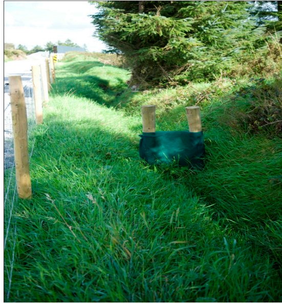
Figure 3-5: Silt trap across grassed swale
