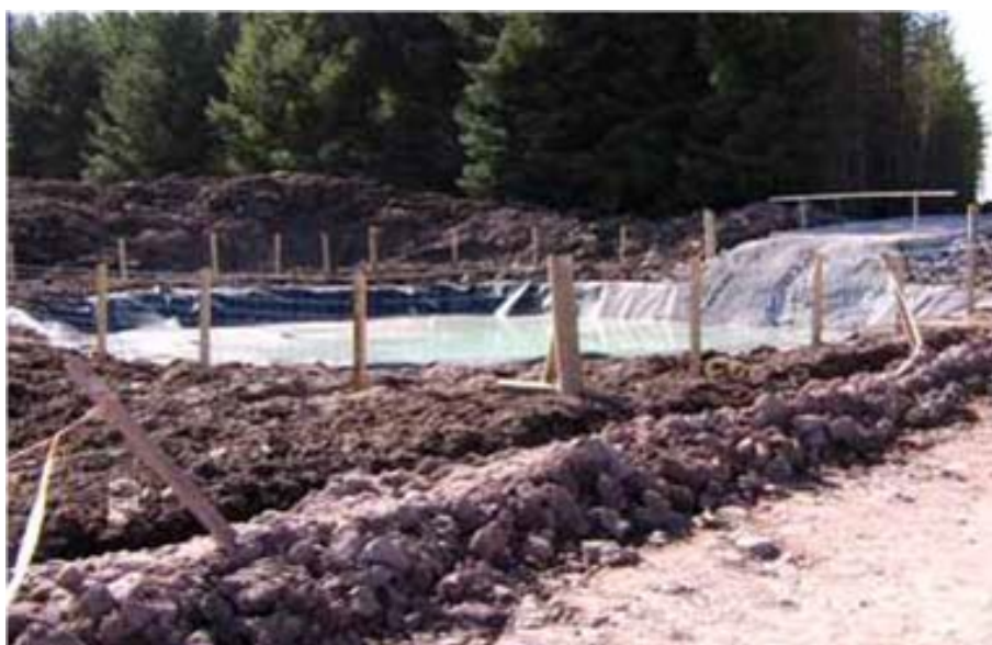
Figure 3-9: Lined Settlement Lagoon for Concrete Washout Facility
