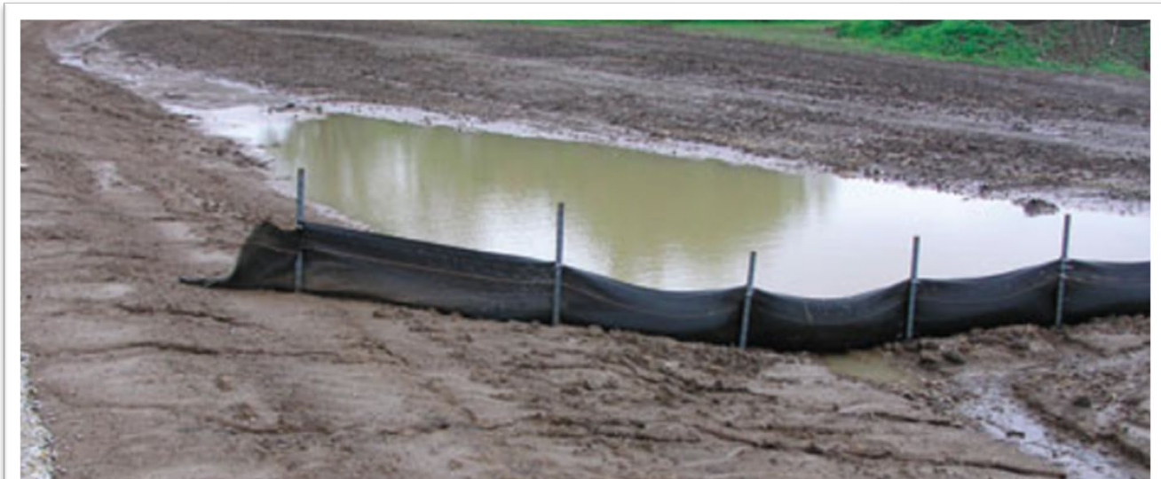
Figure 3-7: Silt Fence
