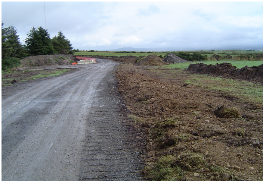
Figure 3-8: Backfill over cable trench
