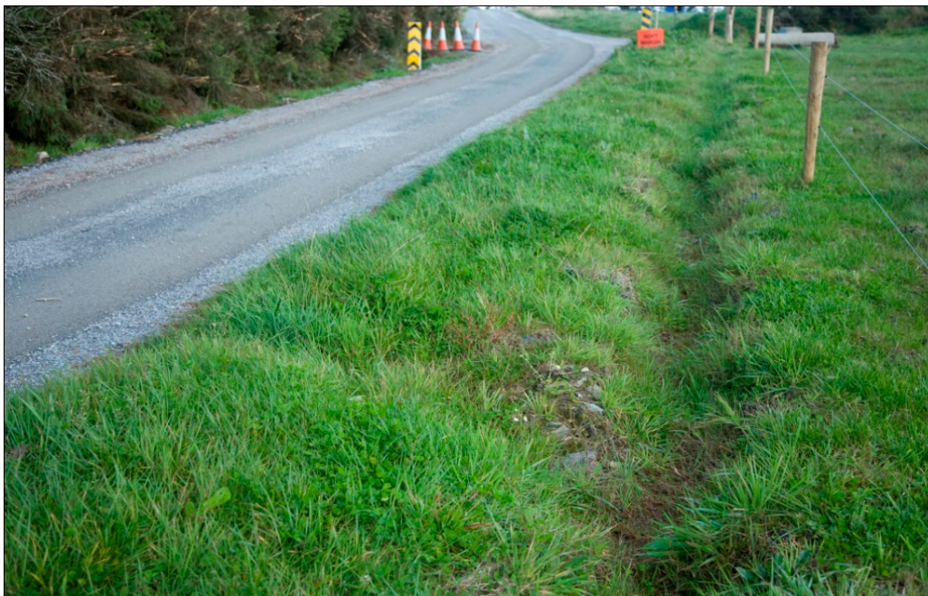
Figure 3-2: Grassed swale along access track
